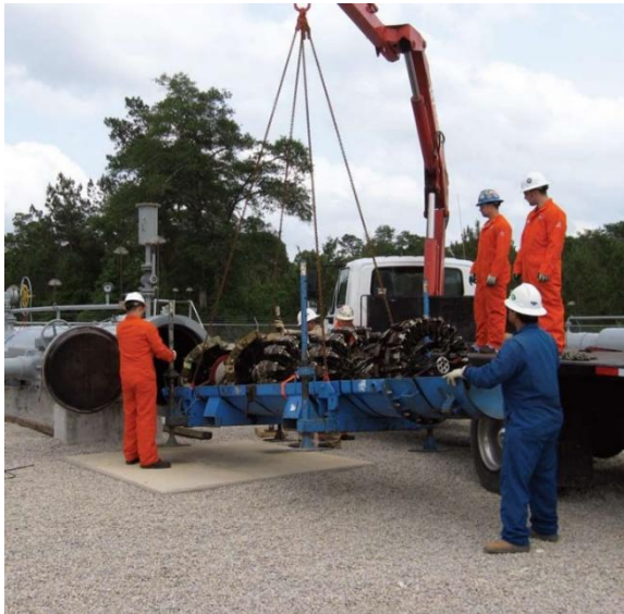
Figure 8: Preparing for ILI launch
