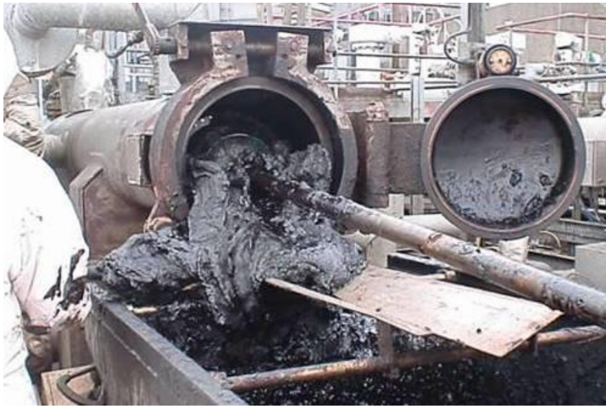
Figure 7: Debris build up within trap as a result of cleaning
